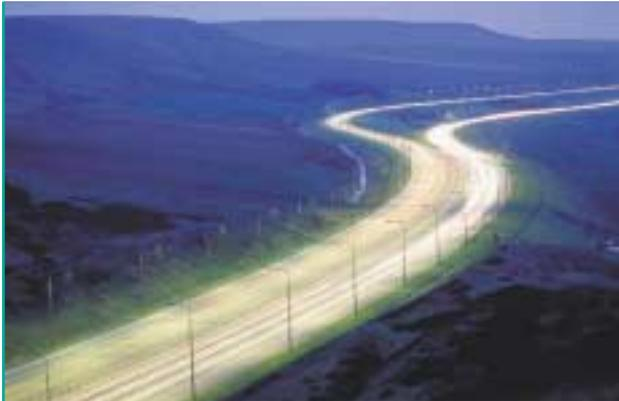
The adverse effects of lighting can be reduced or prevented by using the right technology, design and installation. Road lighting is one of the main problems, and the Highways Agency is now using lighting that focuses the light onto the road surface – as here on the M62 over Saddleworth Moor.
